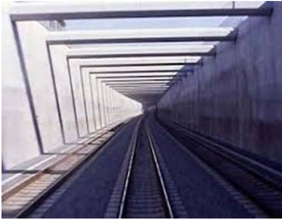
Figure 2: Railroad Trench Source Google Images
