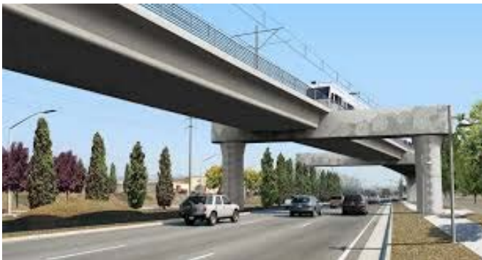
Figure 3: Straddle Bent Source Google Images
