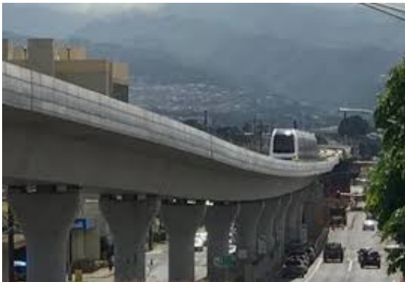
Figure 1: Railroad Viaduct on Median Source Google Images
